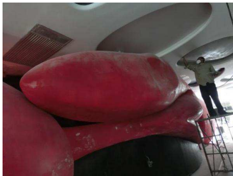
Figure 6. GRG module installation process.
